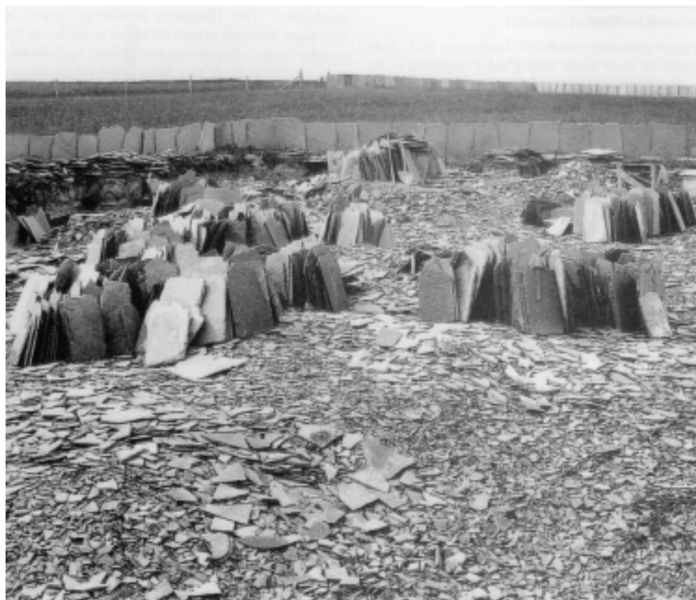
White Moss Quarry, Thurso, c.1910. Thin flags, used as green ornamental stone-slates, are piled ready for export. In the background is an example of a characteristic Caithness 'flag fence' (field wall) with slabs set in the ground on edge in a tight fitting arrangement.
