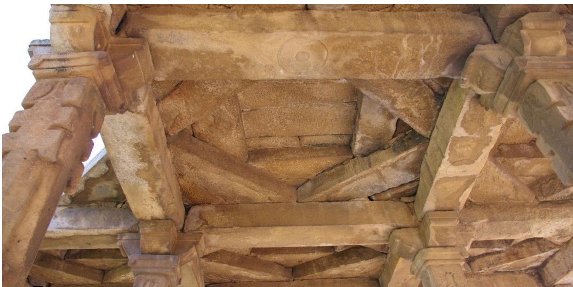
Qutb Minar, Delhi, 1192-1220: Corbelled roof interior
