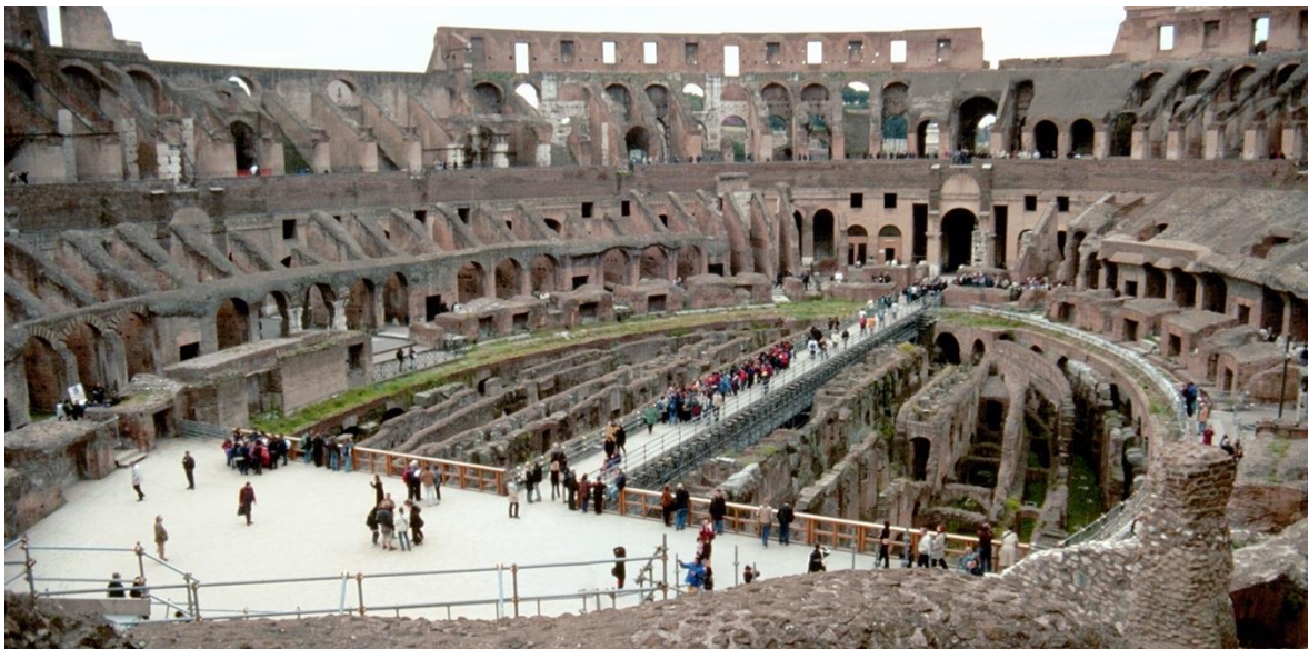
Rome: Making a complex structure safe and accessible
