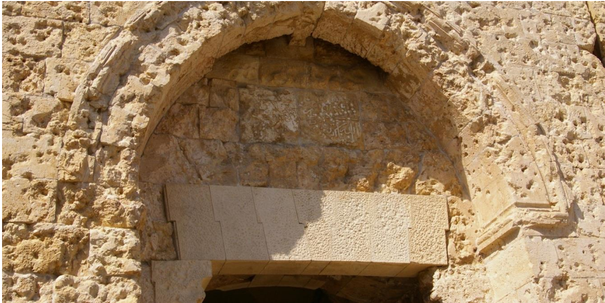
Jerusalem Zion Gate 1540: Structural 2008 crank-jointed flat arch + 1948 war damage
