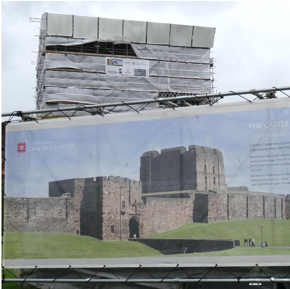
Carlisle Castle: DSC04919 June 2022: Work in progress
