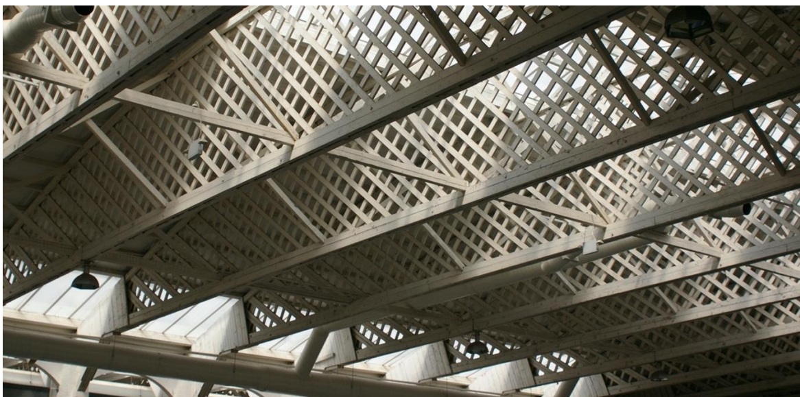
Duxford: General Services Aeroplane Shed 1917 Belfast Truss
