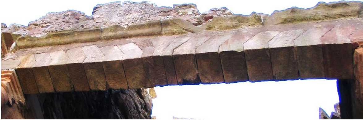
Crank jointed fireplace flat arch
