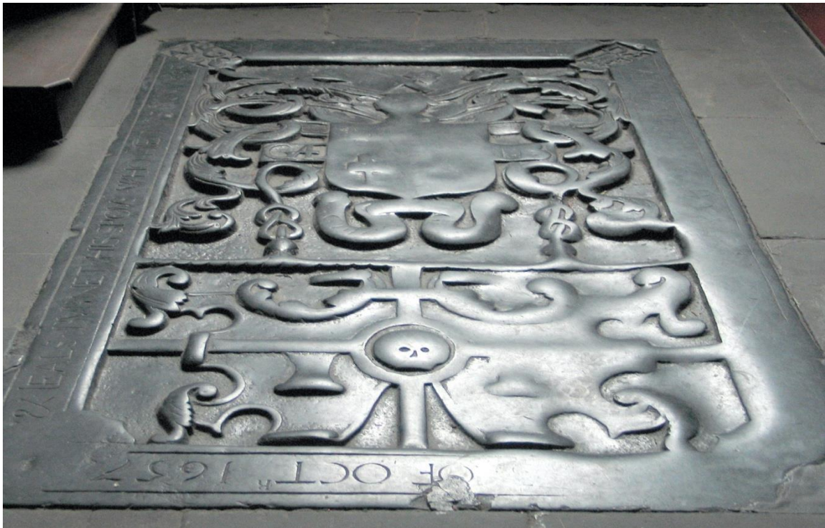
Aberdeen Memorial floor slab: Diagonal footfall wear pattern since 1657
