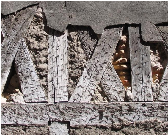
France: Failed render coating over timber framing + Glasgow: Consequences of lack of maintenance and inappropriate previous action
