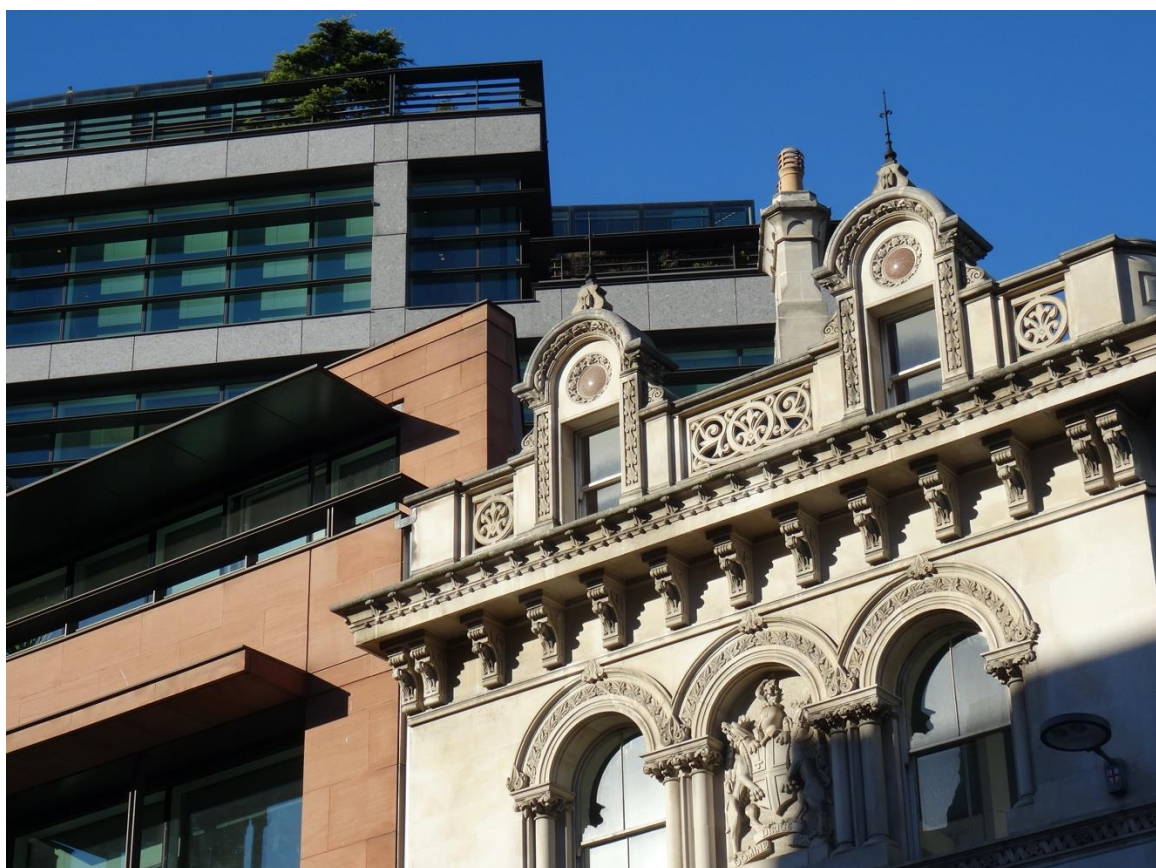
Holborn, London: The design function, fashion, and pattern of buildings change with time
