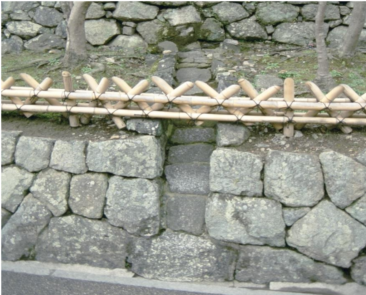
Kiyomozu Dera, Kyoto: Controlled rainwater discharge using indigenous materials
