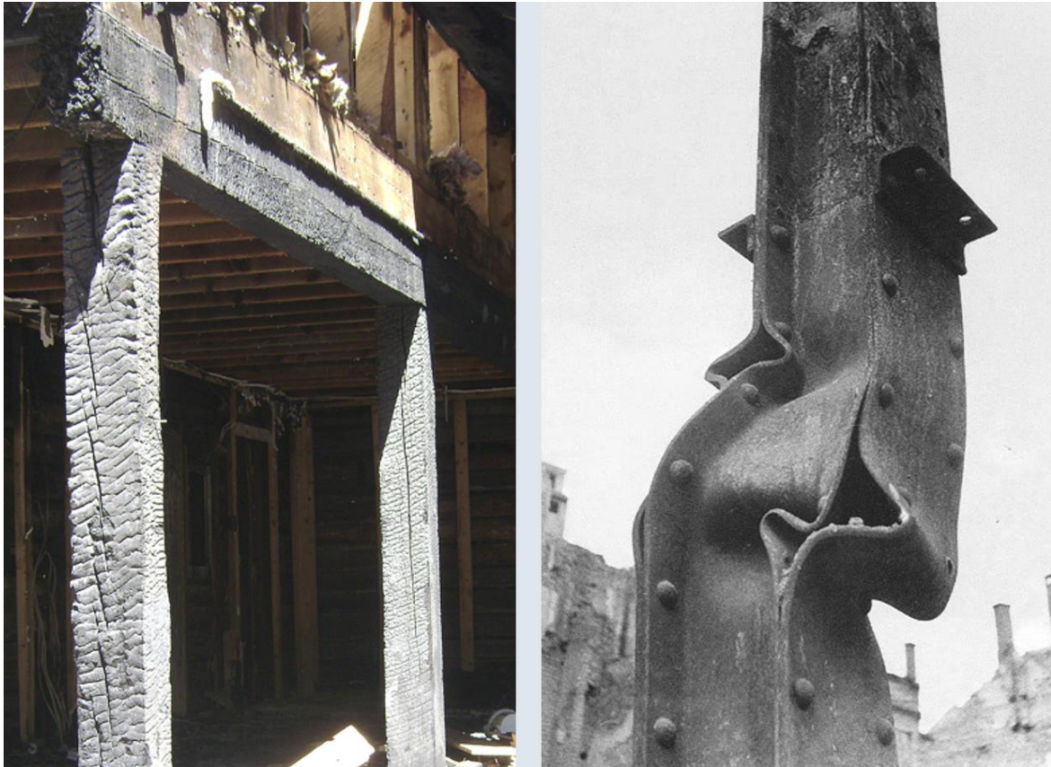
Post fire incident analysis of material performance under stress
