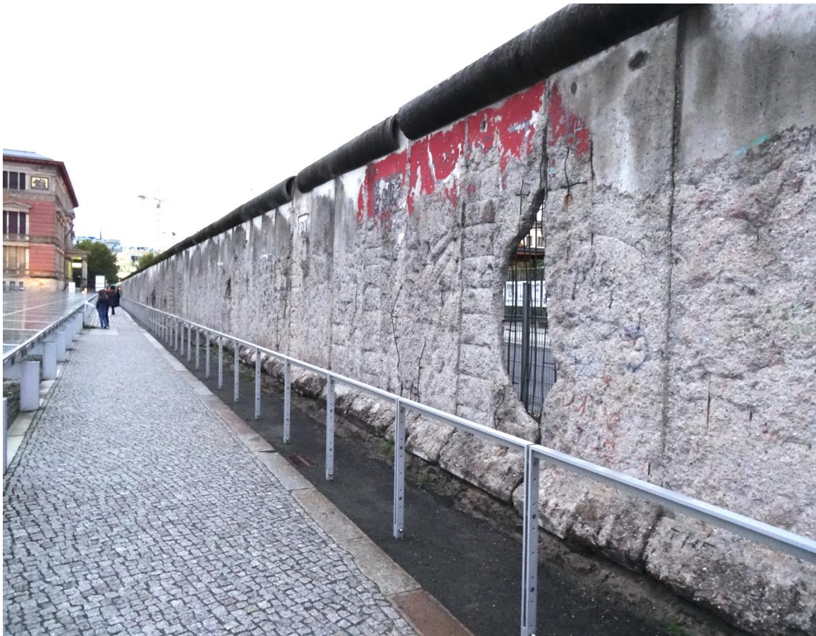
Berlin Wall 1975-80: Original location display section of L-shaped concrete panels
