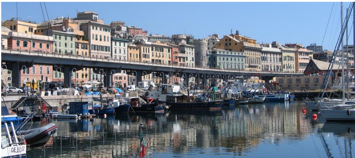
Genoa, Italy: Elevated Harbour Road
