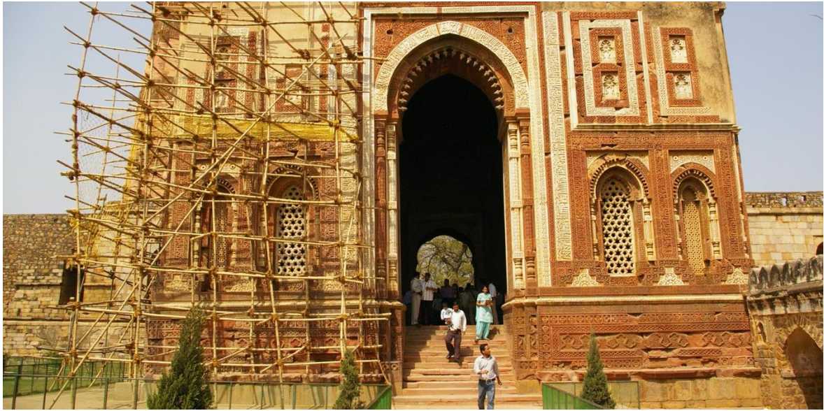
India: Pragmatism in the adoption of local materials for scaffolding
