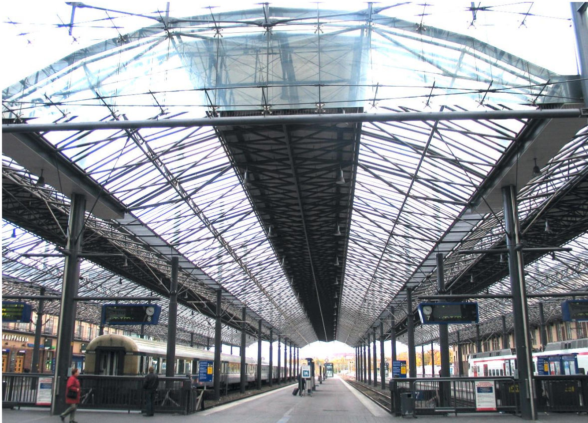
Helsinki's Railway Station: Platform steel framed glass roof structure won in a 1994 design competition and completed in 2001
