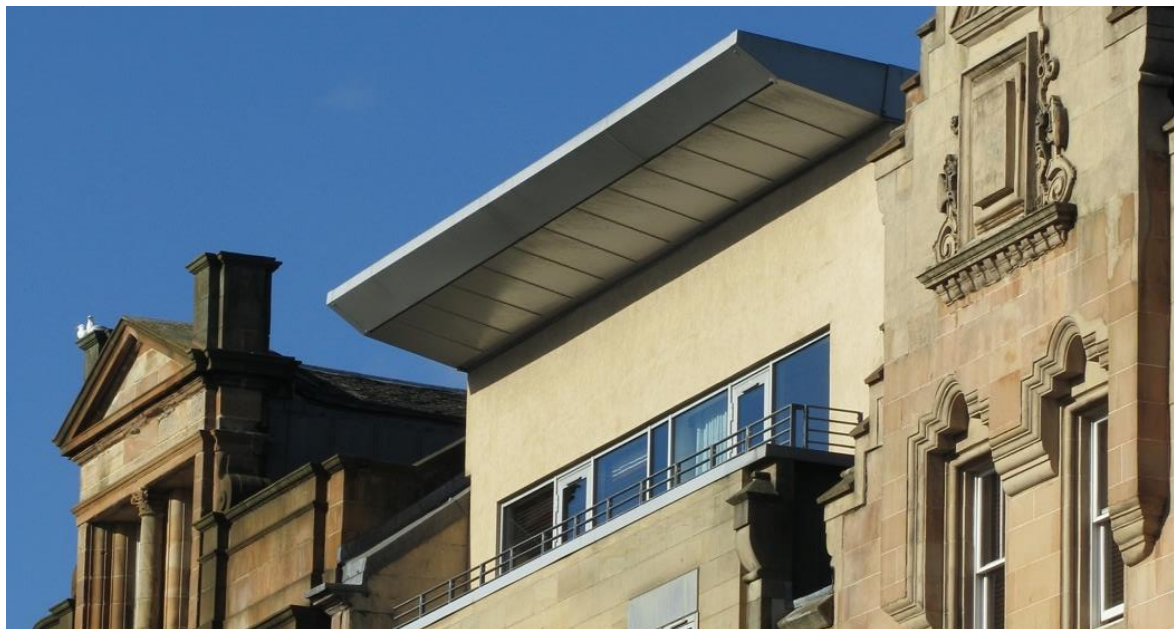
Glasgow: Modern roofscape addition
