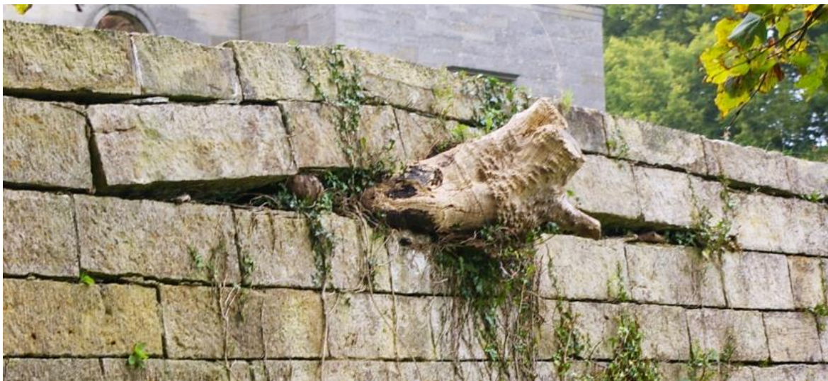
Penicuik: Mature tree root upheaval of masonry
