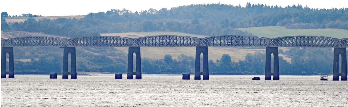
Tay Rail Bridge + Remnants of the 1879 disaster requiring an understanding and diagnosis
