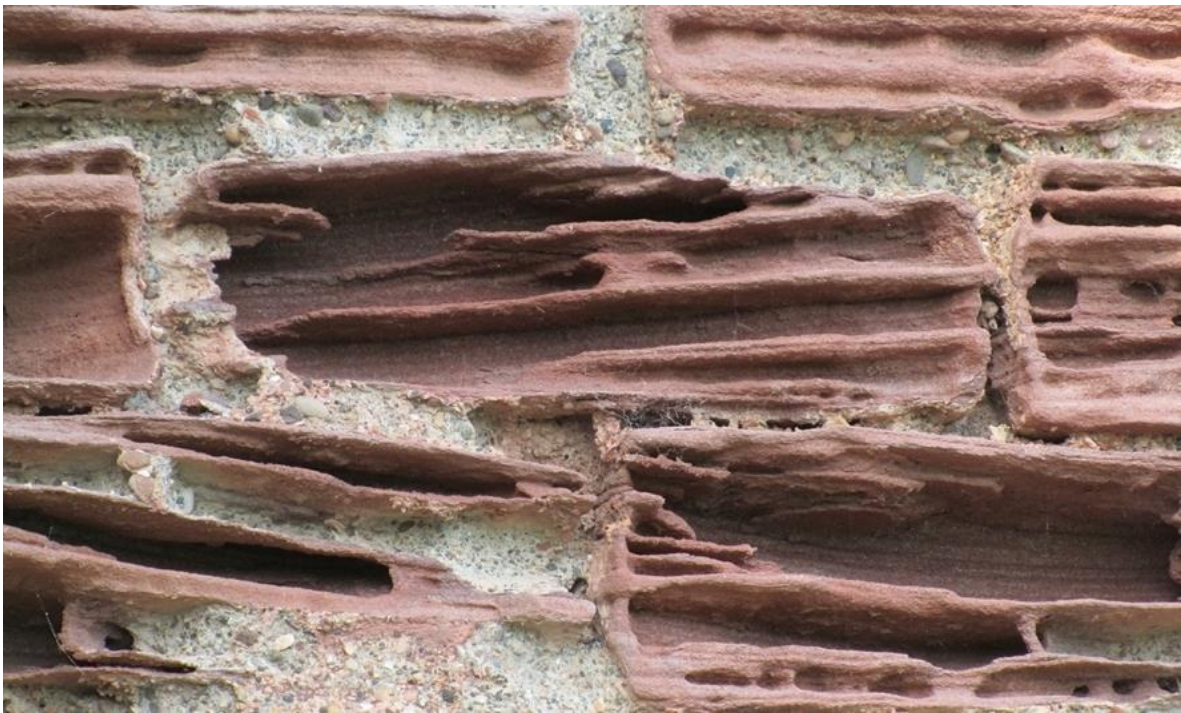
Interaction of hard mortar and variable naturally softer sandstone bedding planes
