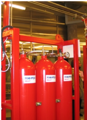
Water mist fire suppression system
