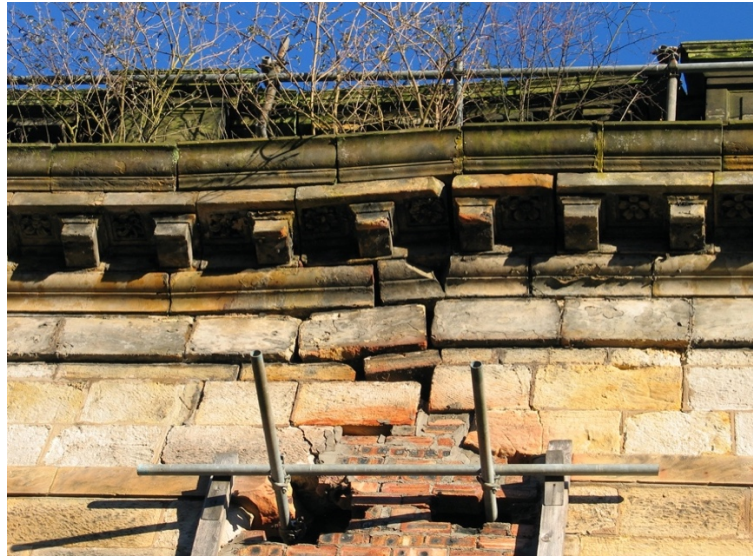
Subsidence caused by poor ground conditions and settlement by abandoned mine workings
