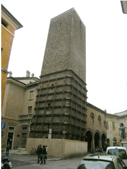
Subsidence caused by poor ground conditions and settlement by abandoned mine workings
