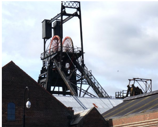
A coal mine pit head winding gear
