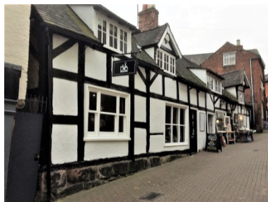
Congleton, a box timber box framed building
