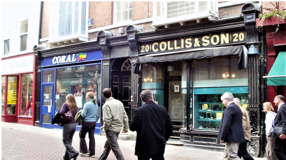
This shopfront in Bury-St-Edmunds was once a single facade. It was visually split into two with imposed corporate identity incorporated on the left. Its natural rhythm is now disrupted: The shopfront on the right is suggested as a better 'conservation' approach to that of the left.
