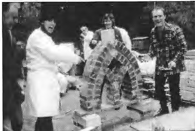
Practice with bedding of building components in lime mortar at the Lime Centre. From left: Mike Adams, Rachel Potzzi, Eugenie Schillig, Andrew Johnson.
