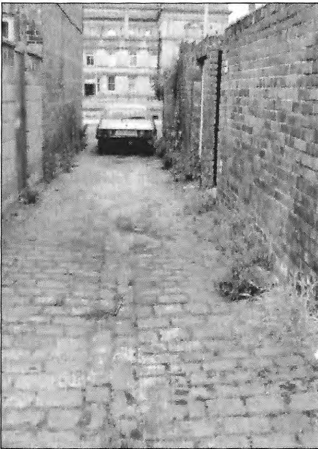
Stone passage before work.
