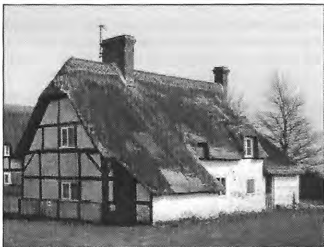
Combed wheat reed, maintained in the traditional manner, with continual patches and repairs. Photograph by courtesy of the NT Kingston Lacey and Corfe Castle estate.
