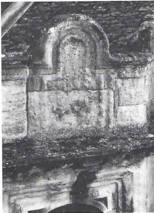
Above: Merton College dormer windows, Oxford BEFORE restoration by Symm & Company Limited.
