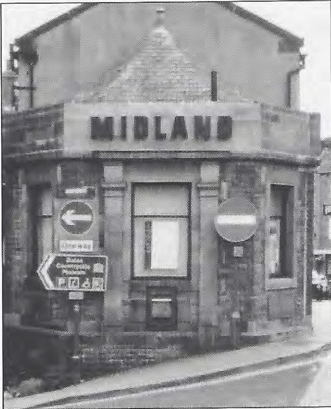
Hawes Bank – the effects of modern street furniture on historic buildings.
