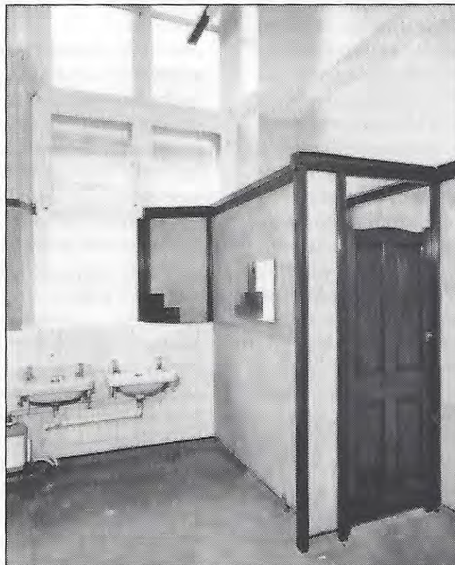
Refurbished Ladies' WC in St Pancras
