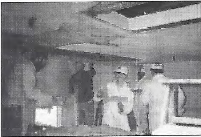
Students in the Historic Plaster Repair workshop at Canterbury Shaker Village, Canterbury, N.H. repair a ceiling in the early 19th century school house.
