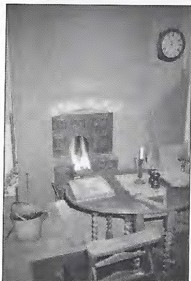
Left: Room 1 – Limewash with red ochre/soot mix, first coat.
