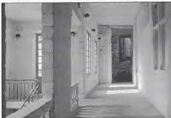
First floor gallery after restoration, L'ecole Avignon.
