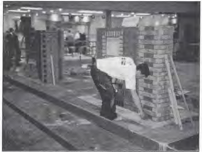
Bricklaying – Skillbuild competition.
