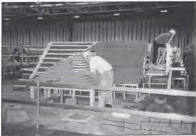
Roof tiling – Skillbuild competition.
