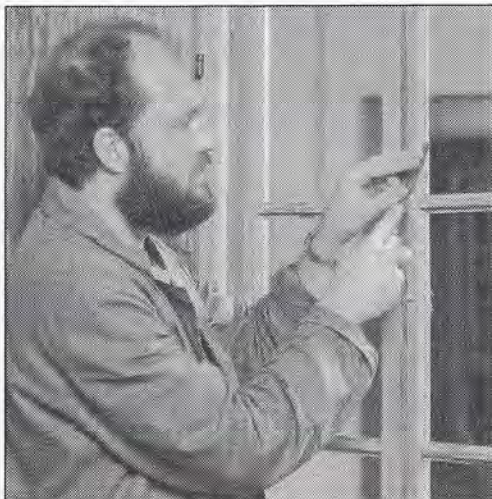
Window repairs at Fulda.
