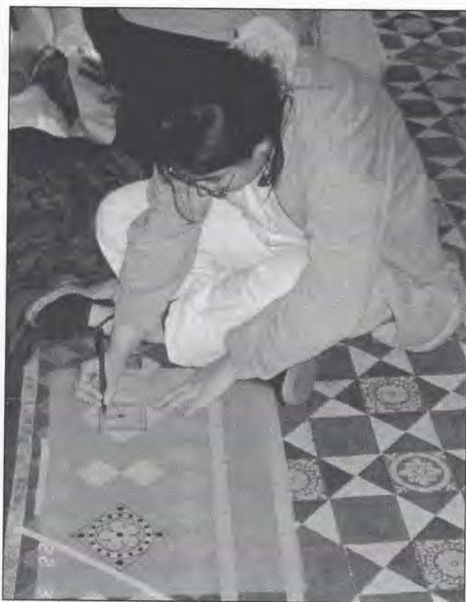
Camden Training Centre student preparing stencil of Minton tiles at St Pancras Chambers.
