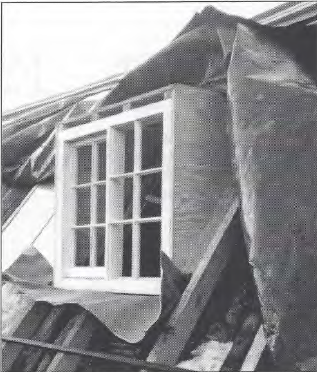
Repaired dormer window.
