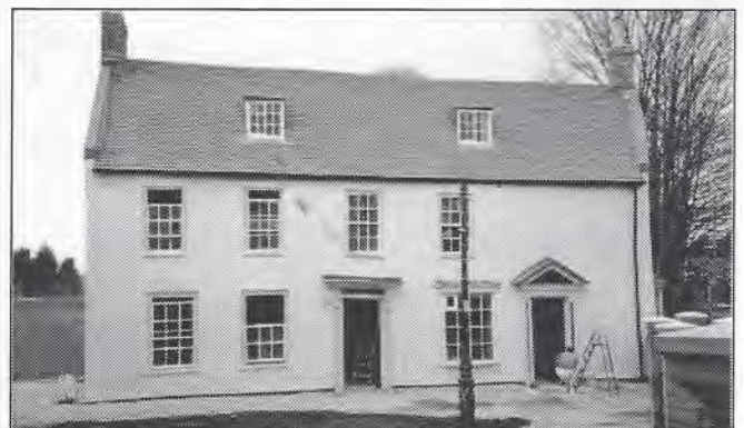
15-17 Bridge Street. Work nears completion.
