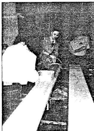
A wooden 'sledge' with a mould cutter inside is pushed along the plank, shaping the plaster.
