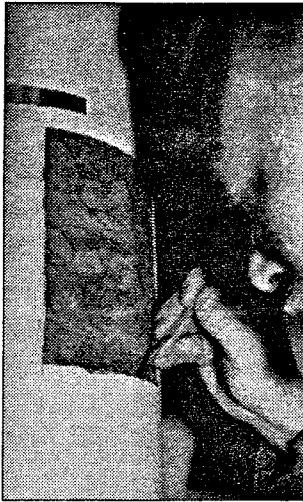
Progressive paint removal on polished limestone columns by student from Lambeth College. See previous page.
