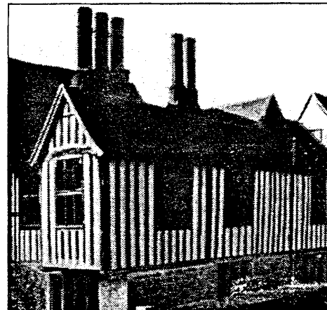
The repair and conservation of oak structure joinery in the north east quarter of Ightham Mote, Kent.
