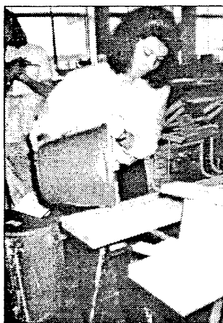
Liquid plaster is poured along the plank.
