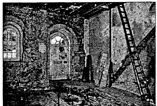
The BCCT offices during repair.
