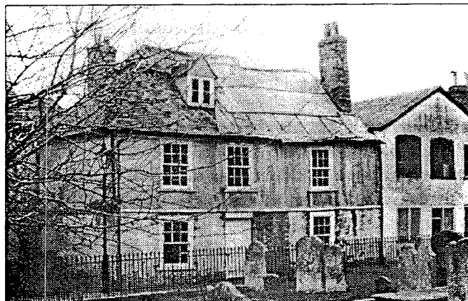
Building proposed for a traditional Timber Frame Repair course
