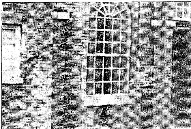
No. 1 The Smithery to be repaired in the Chatham Traditional Brickwork course.
