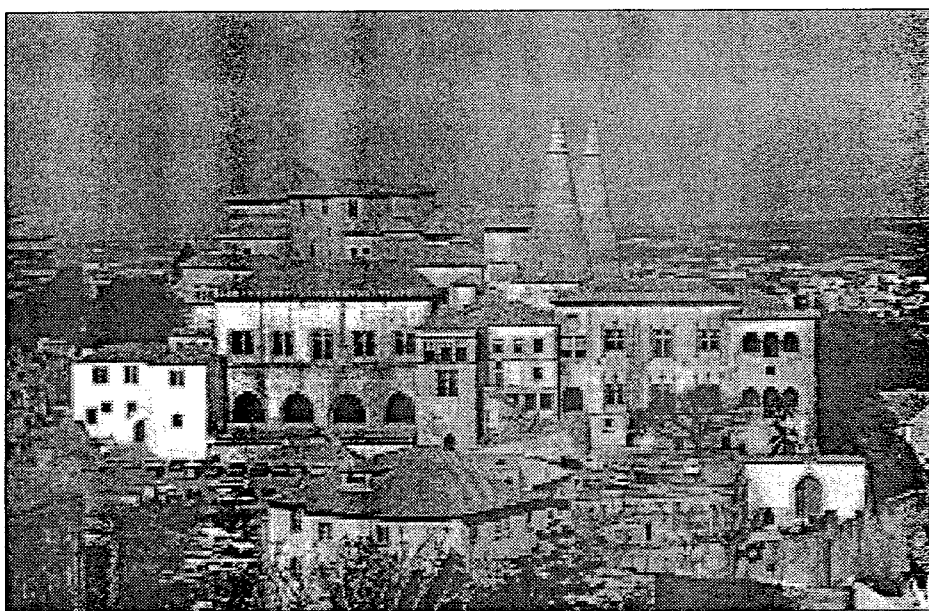
The National Palace at Sintra showing the giant chimneys over the kitchen. See article on Portugal page 15.
