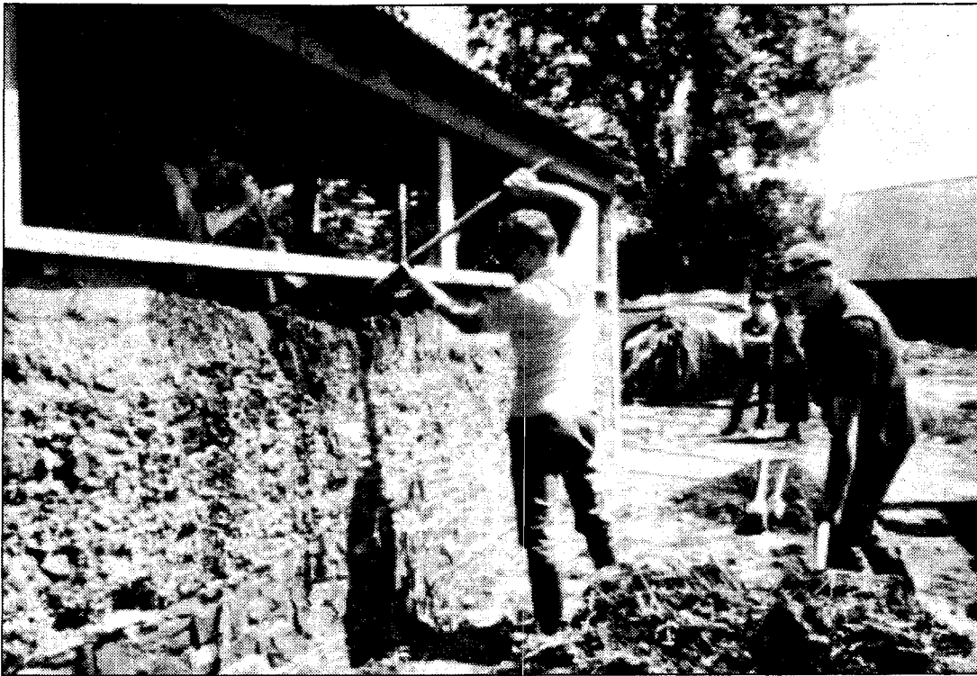
Earth building in action – building a cob wall.
